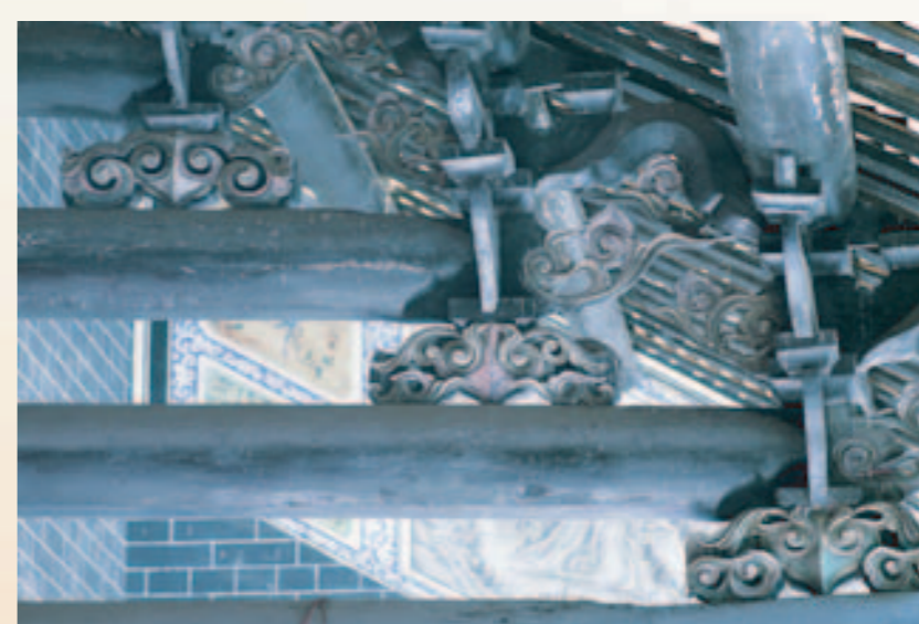
正面鼓台上精緻的木樑架 Delicate wooden truss above the drum platform of the facade
